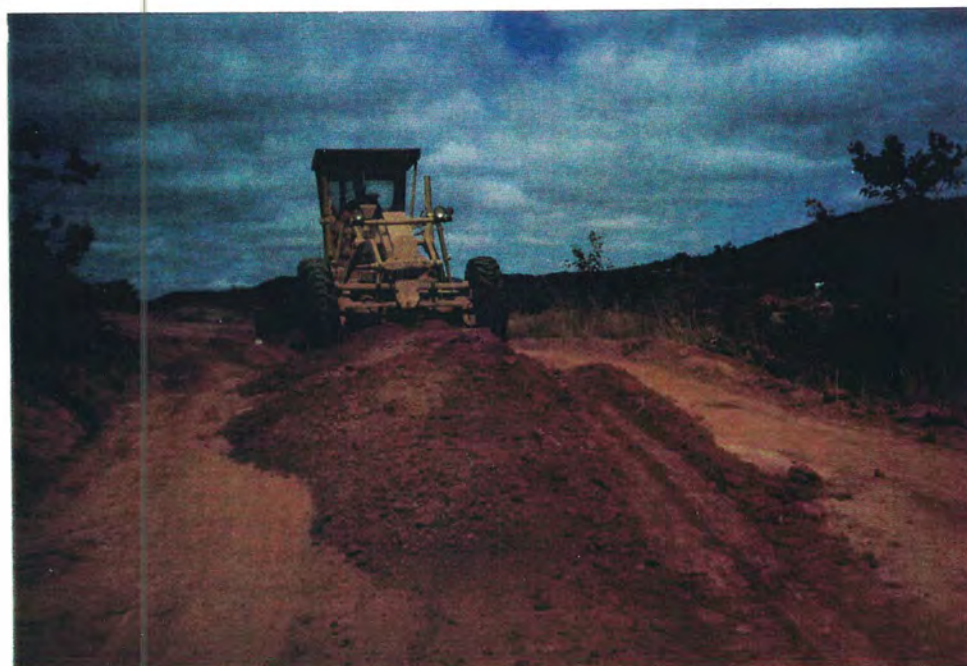
Spreading fill on existing road, Baker Mason IV, Madagascar
