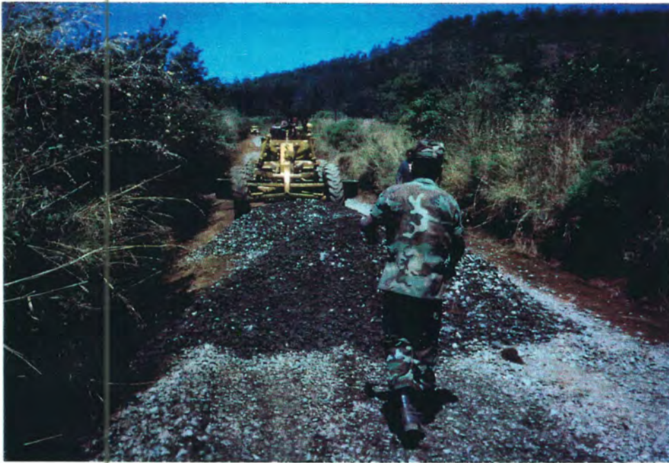
Soldiers spreading gravel on existing road, Baker Mason III, Madagascar
