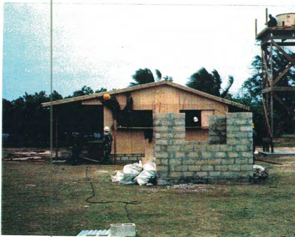
Soldiers installing fascia at Tonga Medical Clinic
