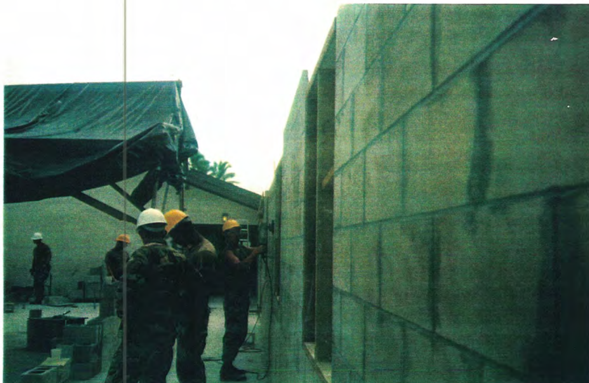
Soldiers finishing CMU wall at George Seitz Elementary School Kwajalein
