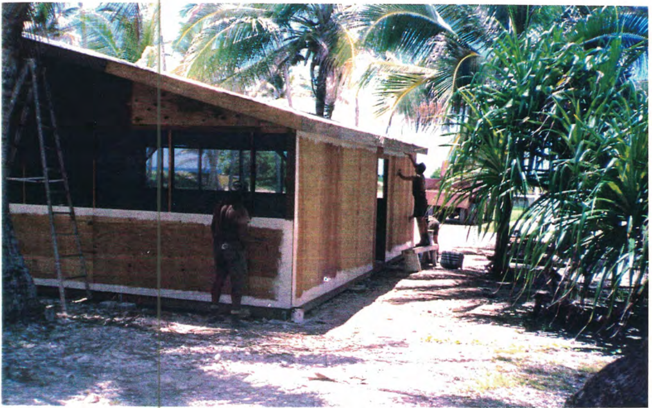
Water purification shed built by CAT Team Kwajalein
