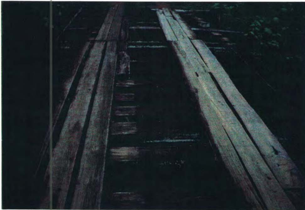
Existing timber trestle bridge in Madagascar prior to our arrival
