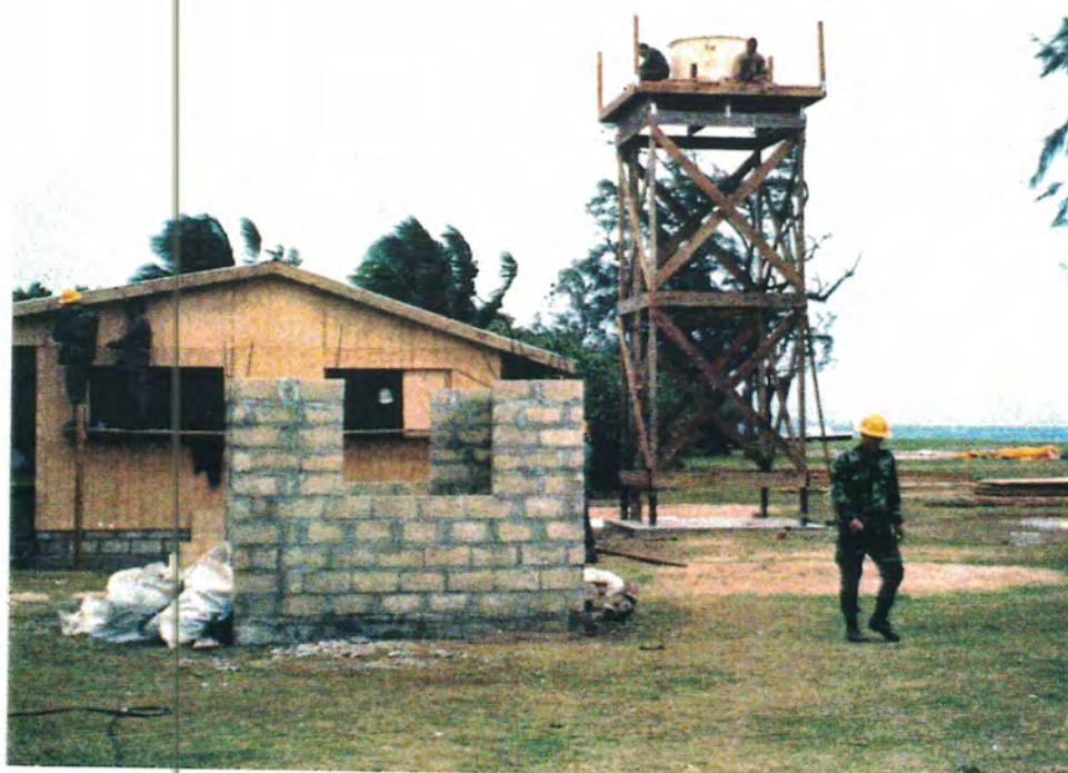
Tongans finishing water tower at Tonga Medical Clinic
