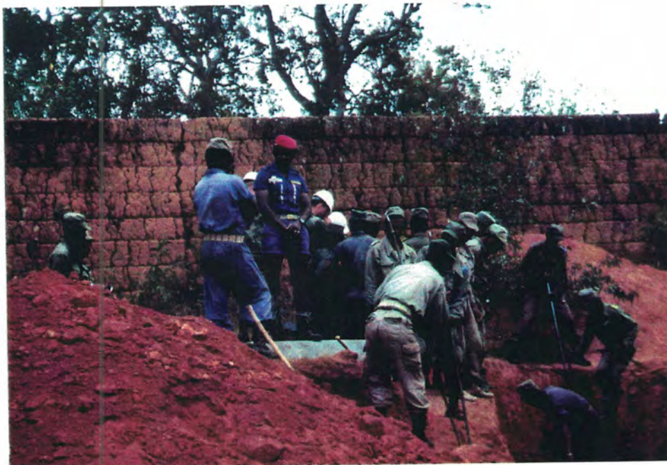
Malagasy soldiers working on installing a culvert, Baker Mason IV, Madagascar
