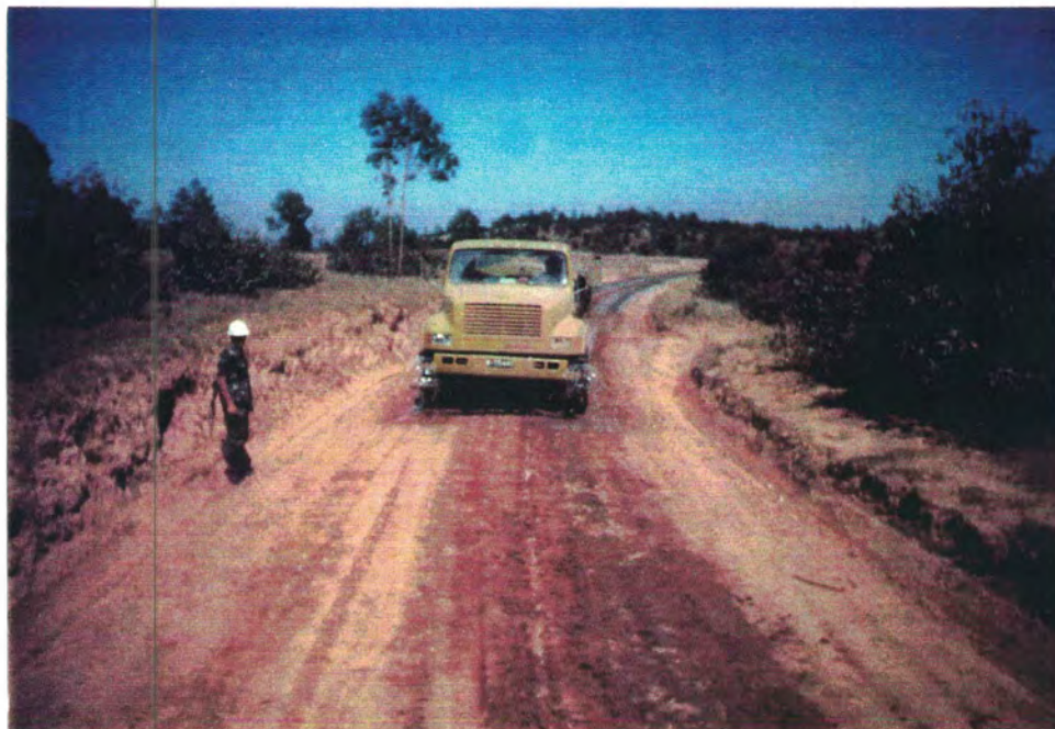
Soldiers distributing water for compaction, Baker Mason IV, Madagascar
