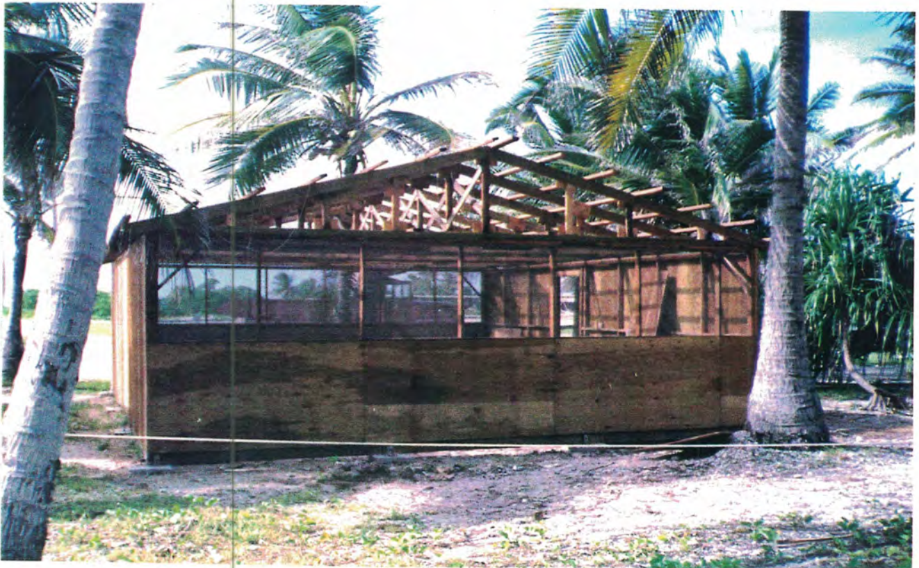
Water purification shed built by CAT Team Kwajalein
