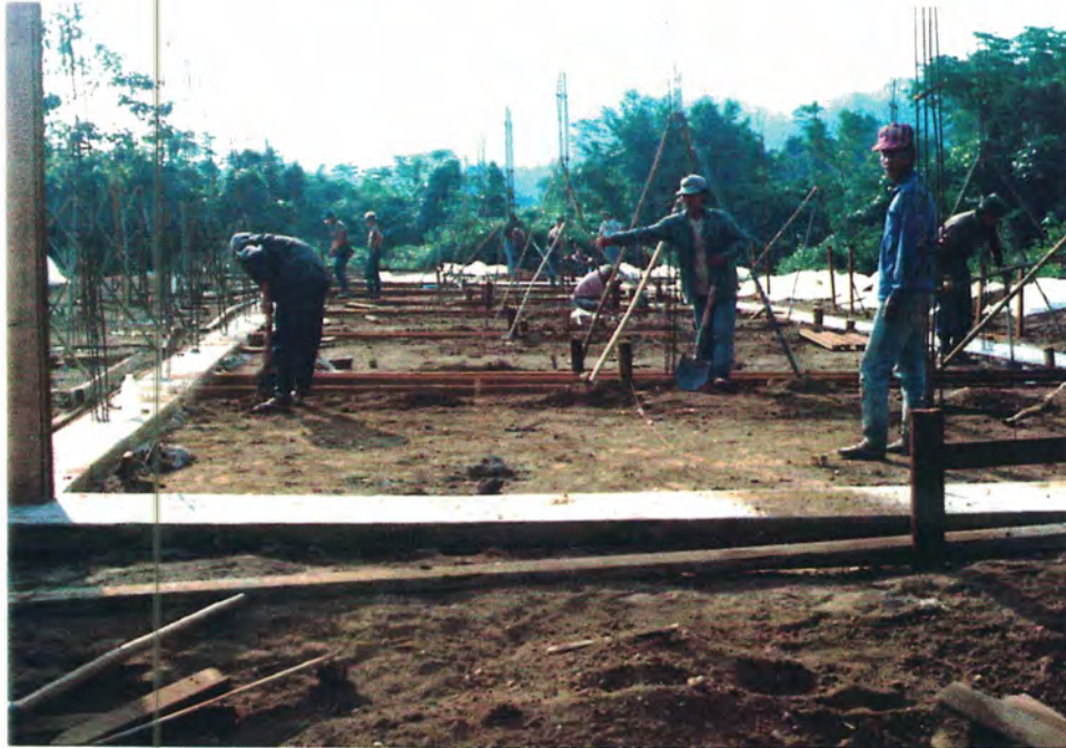
Soldiers preparing foundation for concrete placement, Baker Leader VIII, Laos
