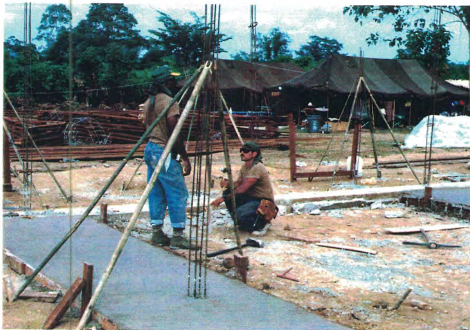
Soldiers preparing form work for columns, Baker Leader VIII, Laos
