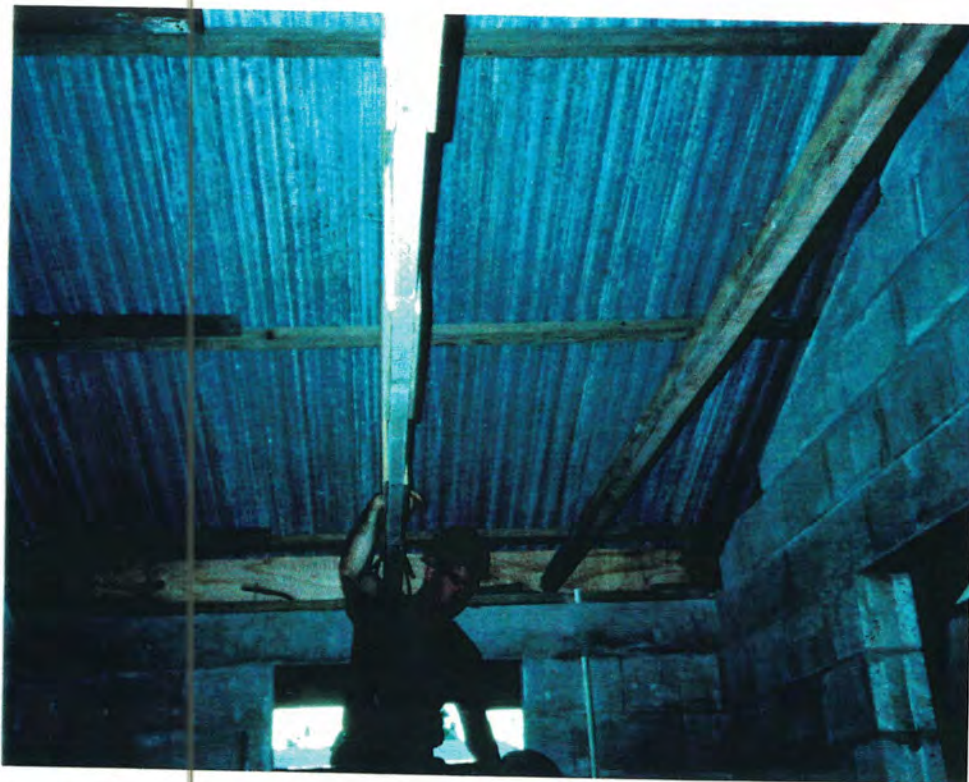
Placing electrical wires & fixtures in an office extension completed by CAT Team Kosrae
