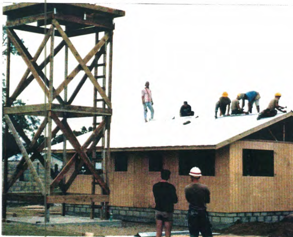
Soldiers and civilians installing corrugated roofing at Tonga Medical Clinic
