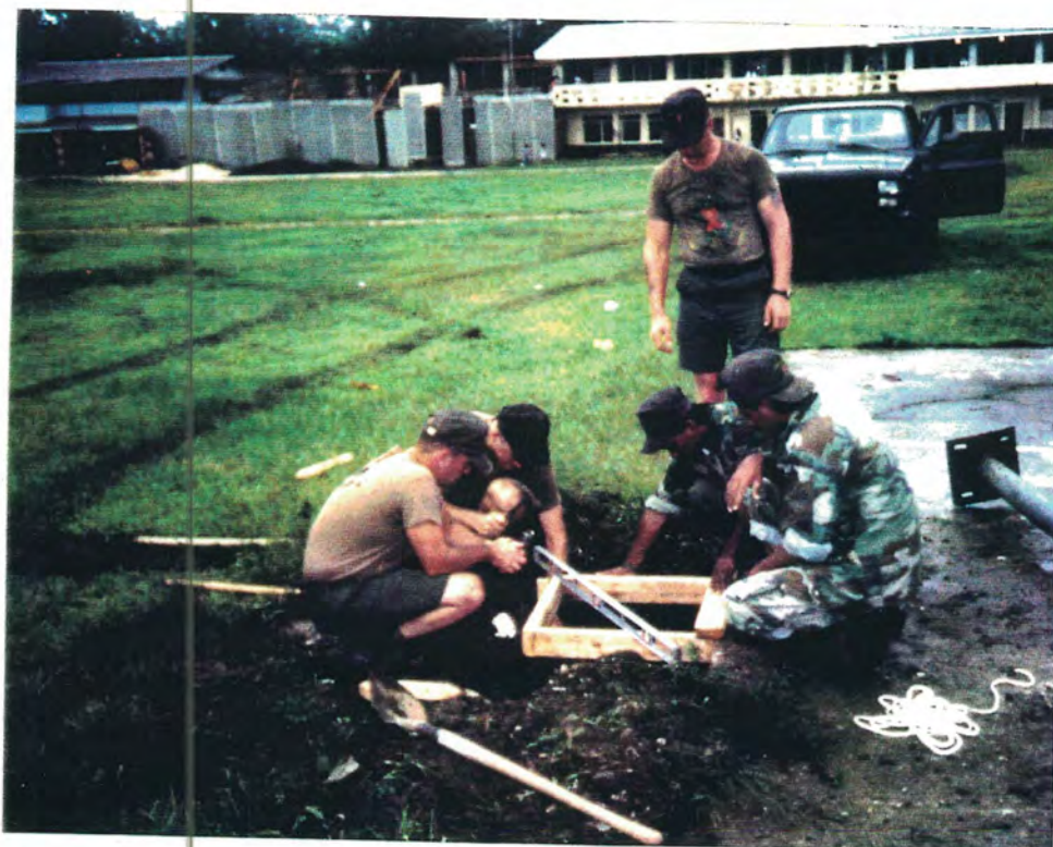
Soldiers placing formwork for basketball backboard CAT Team Kosrae
