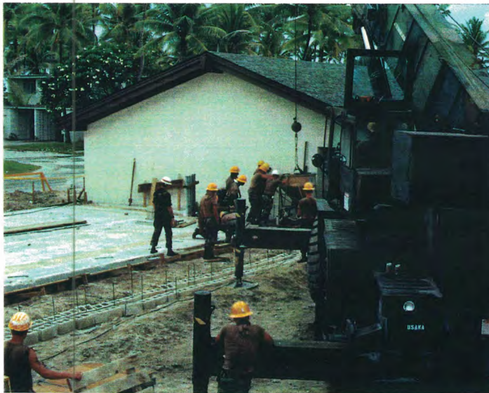
Soldiers placing footers at George Seitz Elementary School Kwajalein
