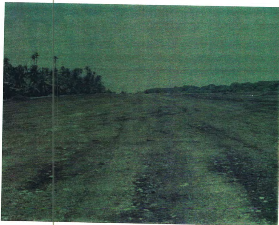
Completed runway CAT Team Kwajalein
