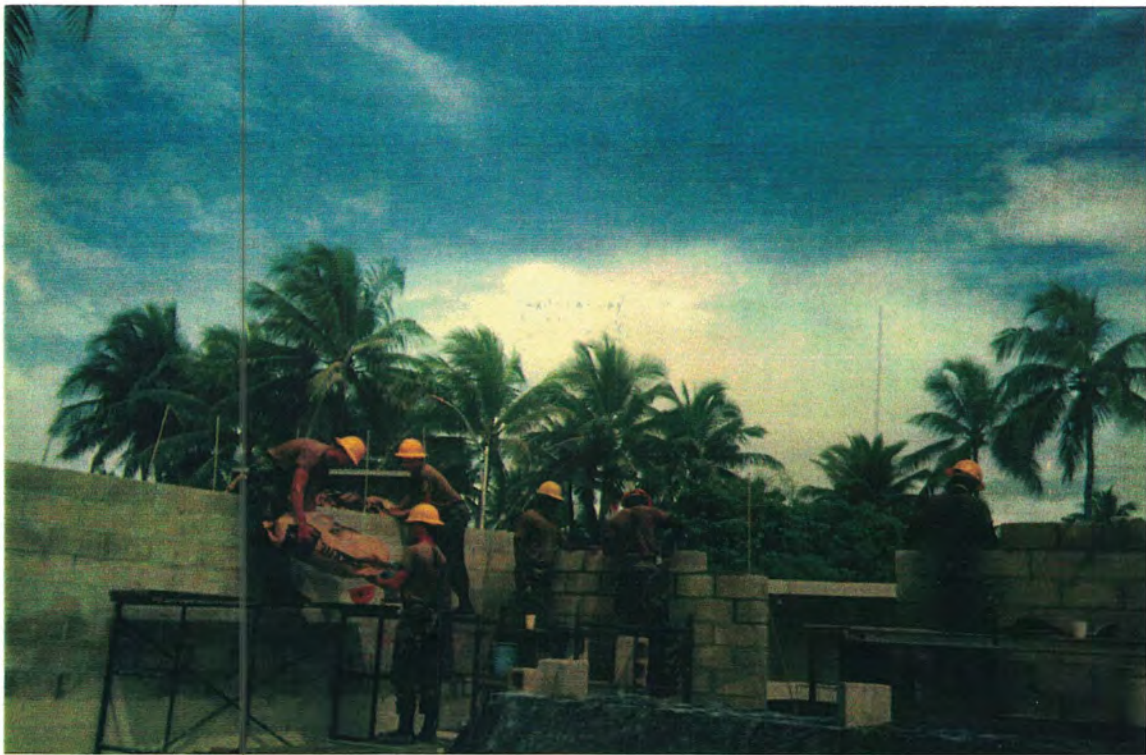
Soldiers placing CMU at George Seitz Elementary School Kwajalein
