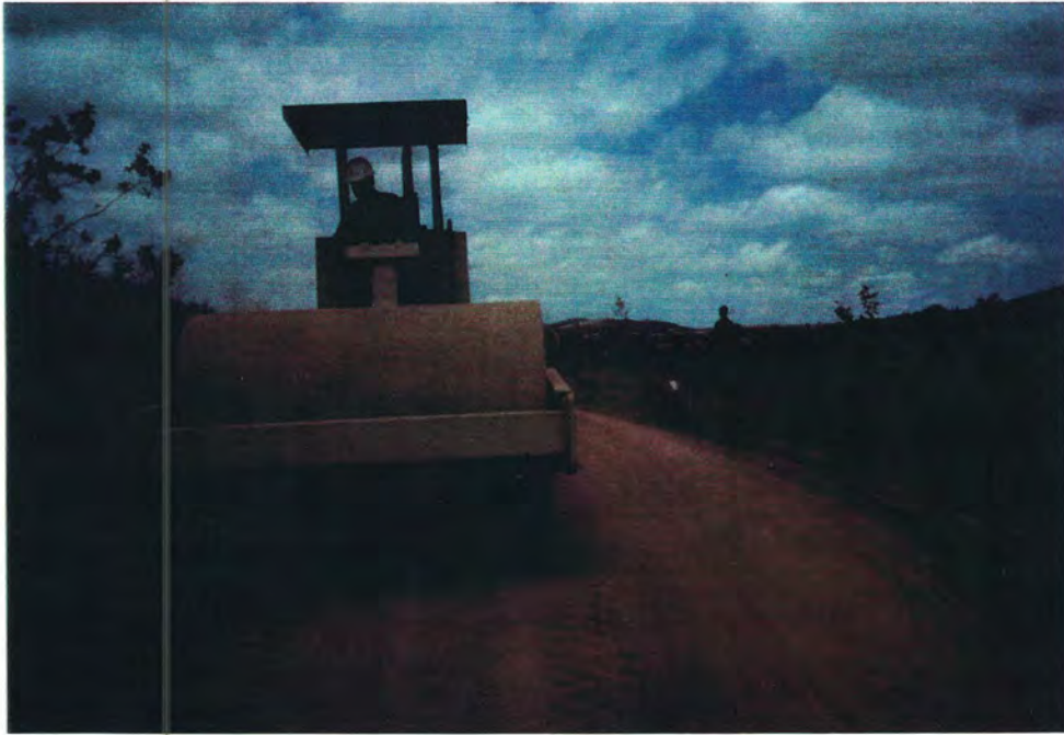
Soldiers compacting gravel on existing road, Baker Mason IV, Madagascar
