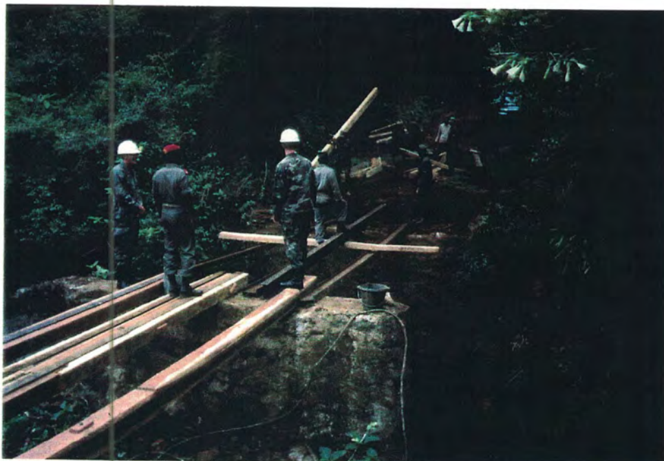
Rebuilding of timber trestle bridge, Baker Mason III, Madagascar
