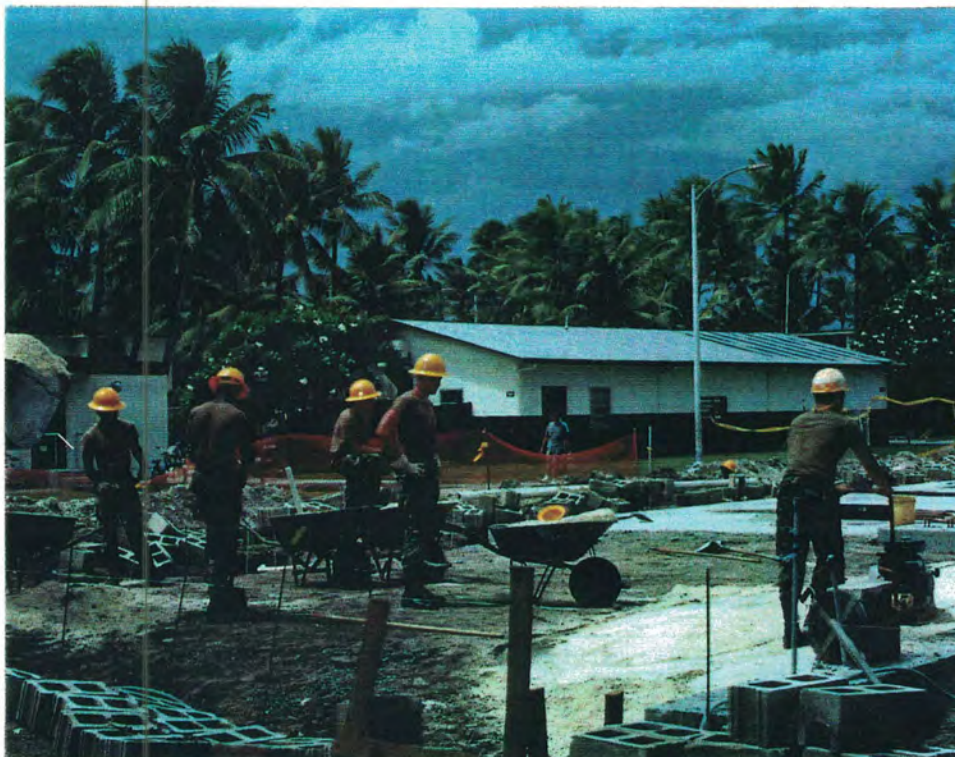
Soldiers preparing to lay block at George Seitz Elementary School Kwajalein
