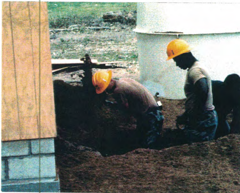
Soldiers excavating for septic tank at Tonga Medical Clinic
