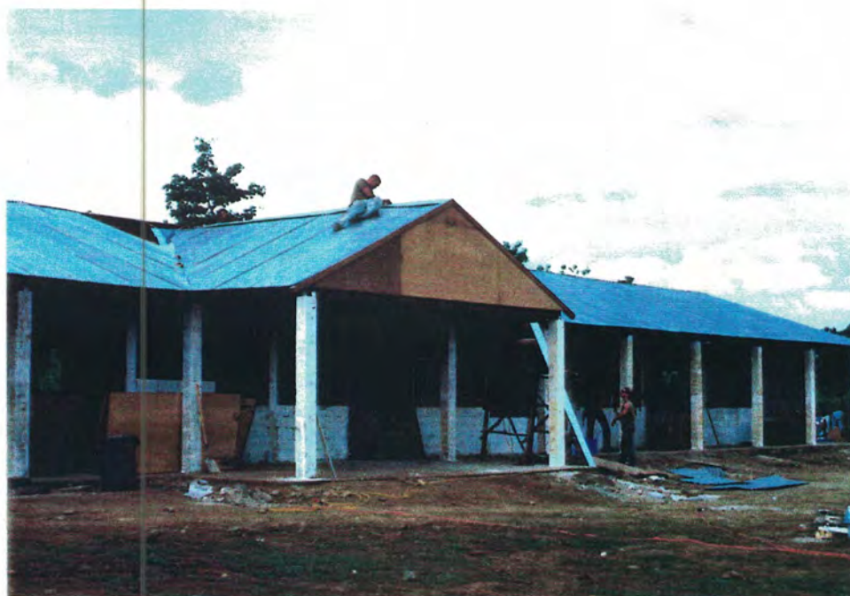
Soldiers finishing corrugated metal roof, Baker Leader VIII, Laos
