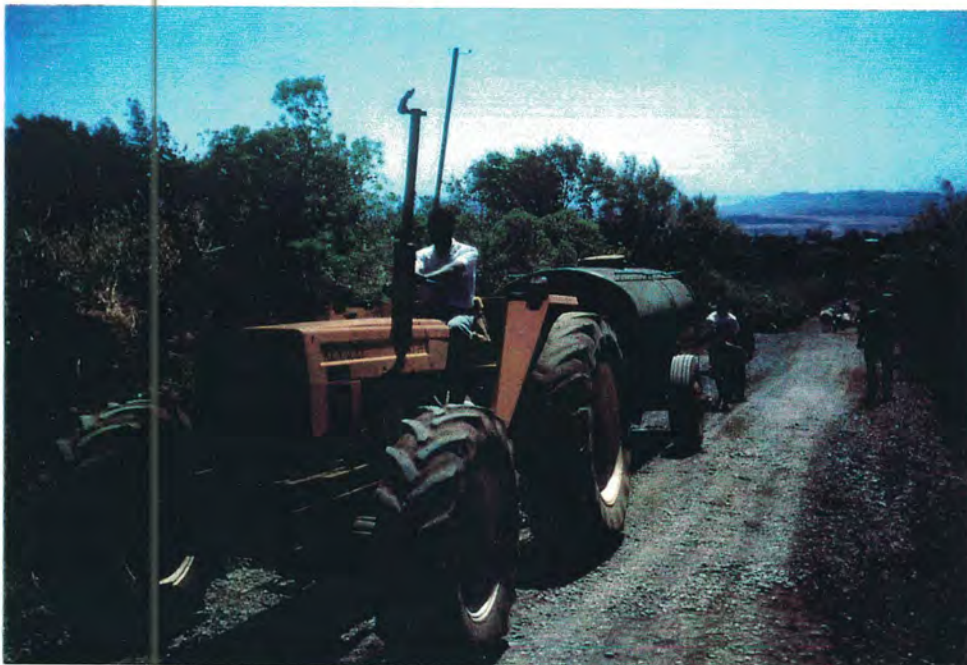
Civilians distributing water for compaction, Baker Mason III, Madagascar
