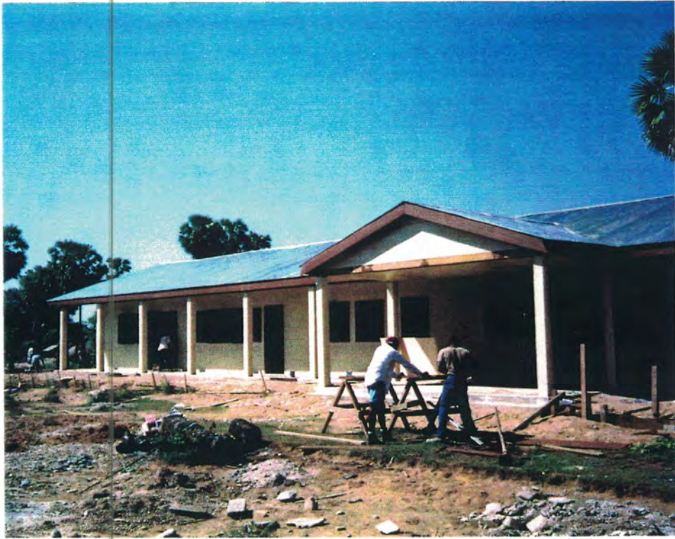
Soldiers applying finishing touches, Baker Leader VII, Laos
