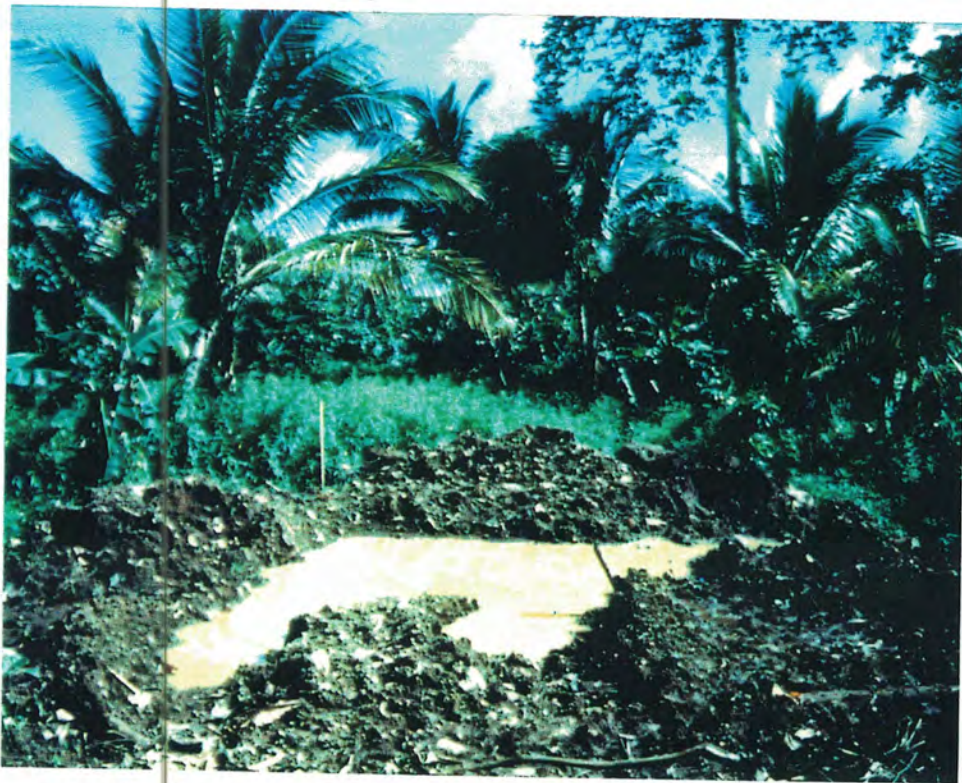
Clearing and grubbing for new travelway CAT Team Kosrae
