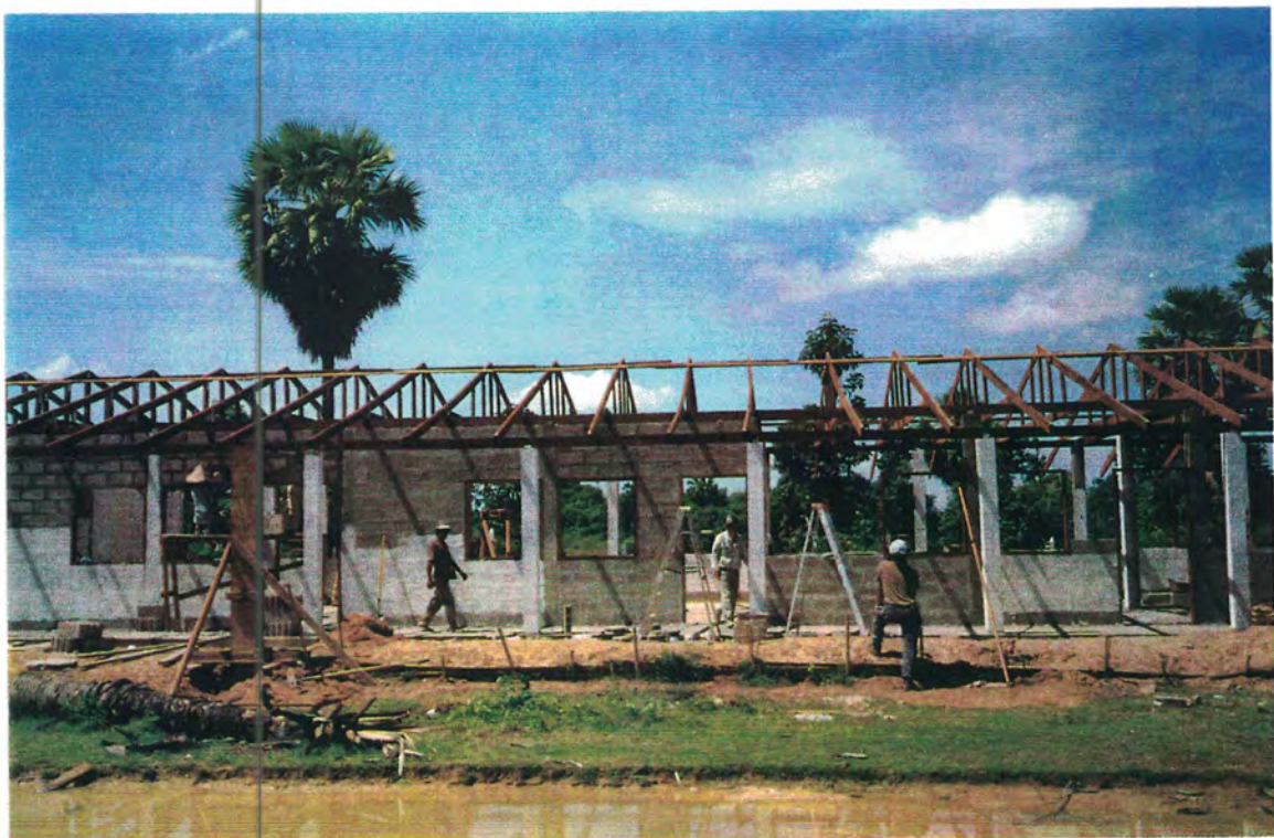
Soldiers preparing roof for decking, Baker Leader VII, Laos
