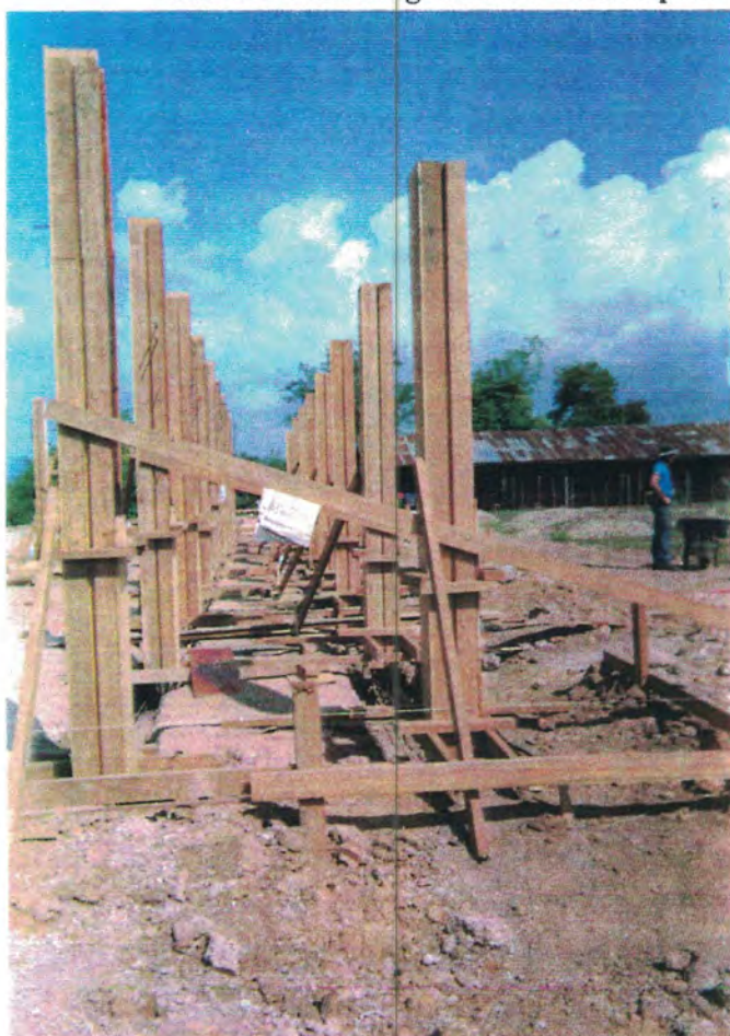
Mixing concrete with concrete mobile and column placement, Baker Leader VI, Laos
