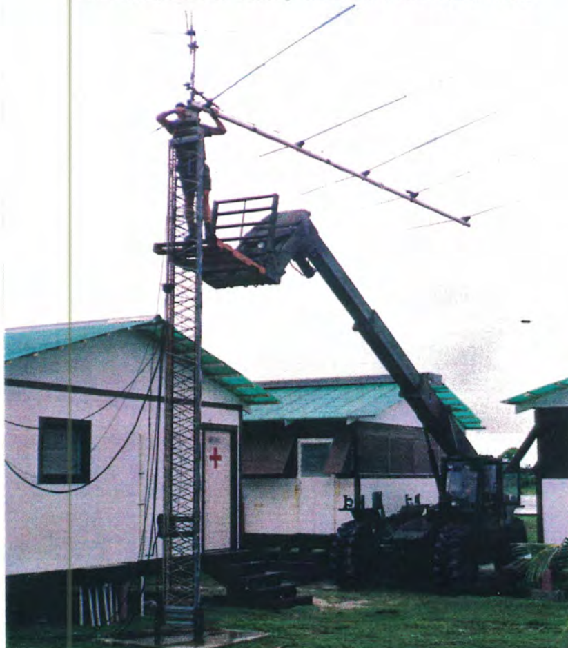
Erecting an antennae for CAT Team Kwajalein
