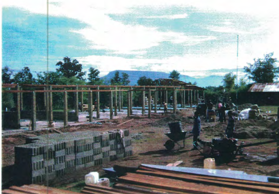
Beam and rafter placement, Baker Leader VI, Laos
